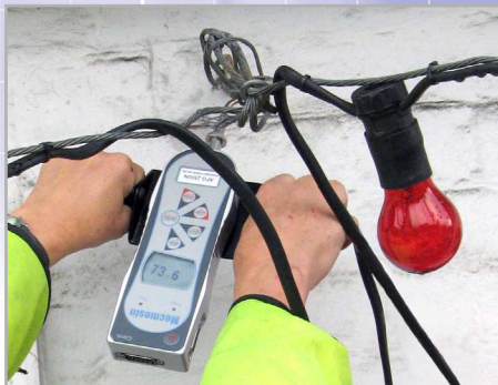
Pull test on anchorage points
